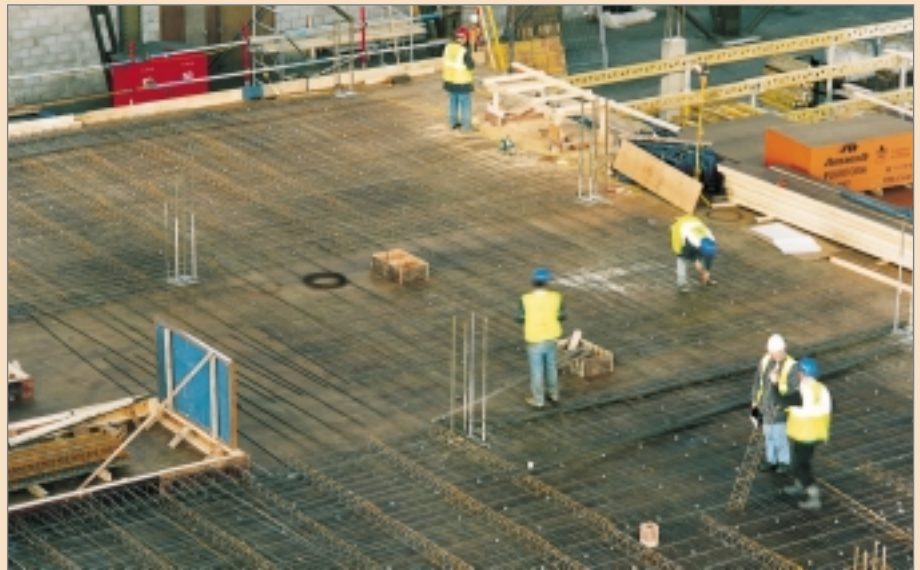
Figure 2: The reinforcement to Floor 1 at Cardington during construction
