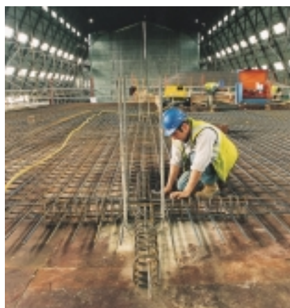
Figure 7: ACI shear stirrups were prefabricated at Cardington
