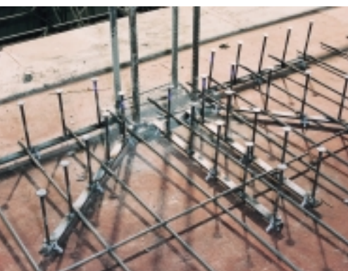
Figure 5: Stud rails at Cardington
