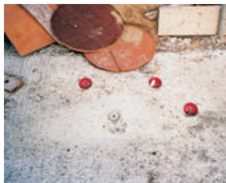
Figure 3: Floating cups grouped at edge of pour. One has already been pulled out.
