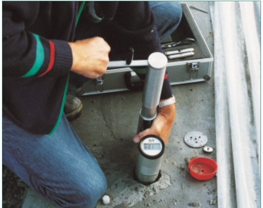
Figure 1: the Lok-test jack in position.
